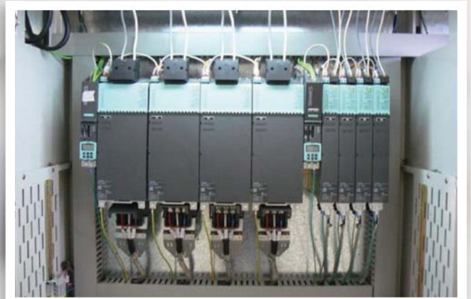
AC & DC Variable Speed Drive Panels
